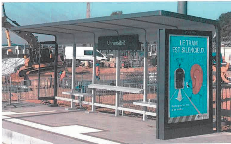
Abri de station
