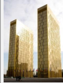
Civil Construction & Infrastructure Projects
